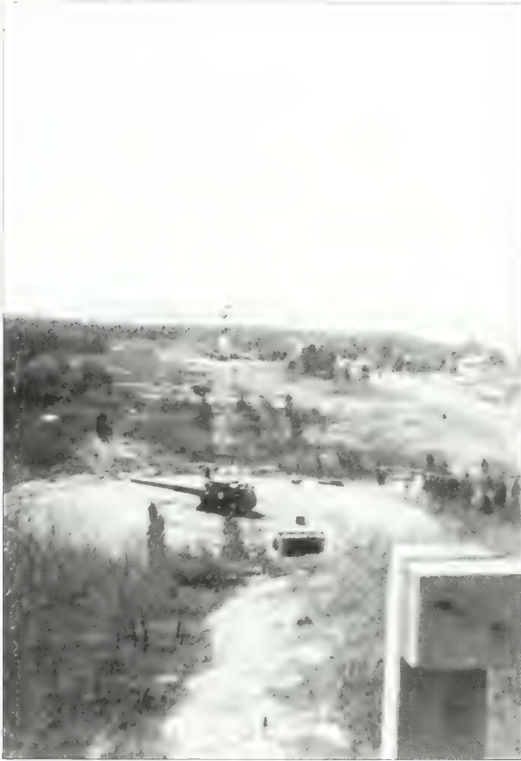
Figure 5.79. View looking north of gun emplacements at Batteries Kingman and Mills. Prior to 1941, the guns were emplaced on open platforms that permitted 360-degrees of rotation and firing. The north emplacement at Mills is in the foreground and beyond that the south emplacement at Kingman (GATE 938).
